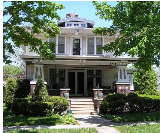
844 E. Pacific, corner of E. Pacific and N. Rankin in Appleton's current 3 rd Ward (photo courtesy of Donald Elston)
